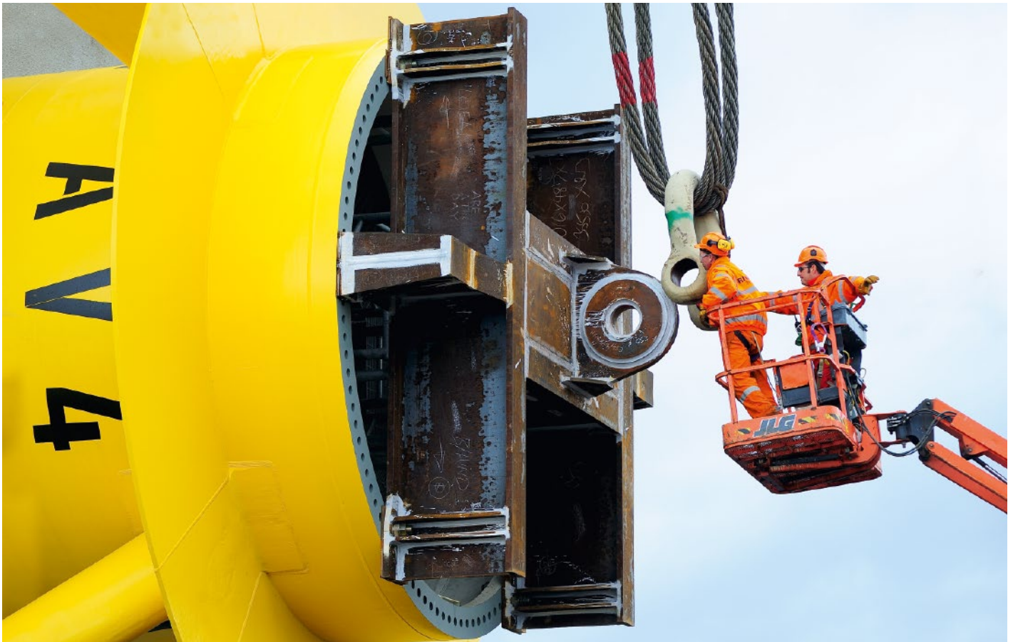
CLOSE INSPECTION even of the large components.
